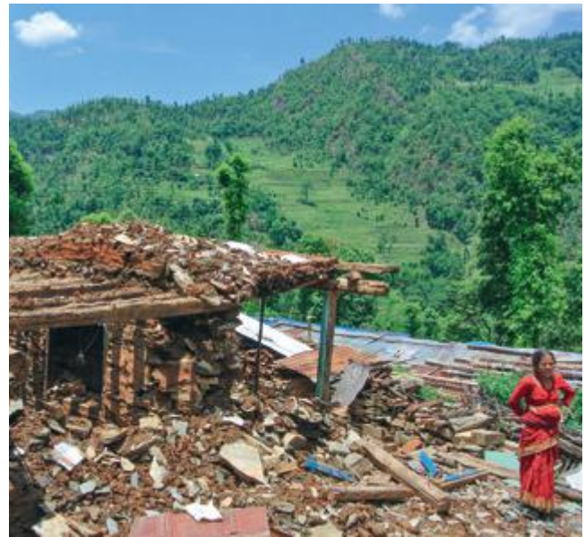
Almost a million houses were destroyed by the earthquake in Nepal, most of them loosely fitted with traditional materials
