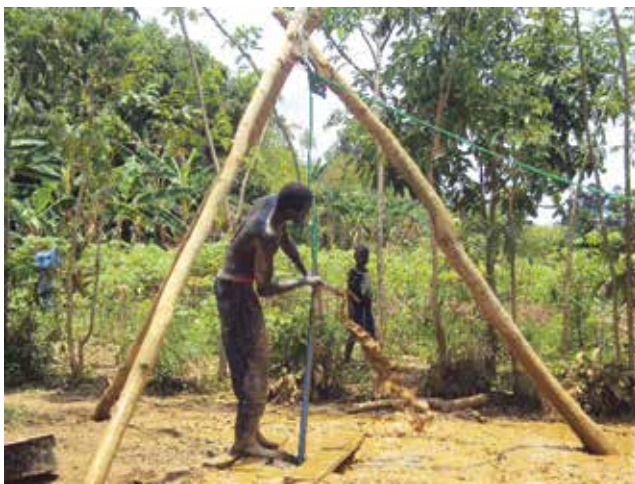
Manual drilling in process
