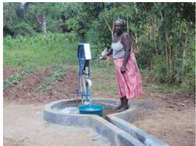
A completed low cost well fitted with a rope pump
